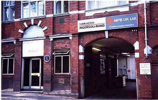
Fig. 188 The Sunbeam factory, 1899-1935.
