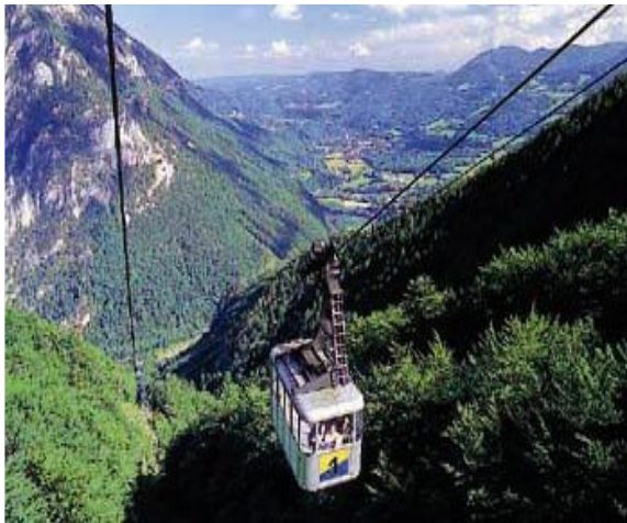
Fig. 60 Raxbahn cable car above Semmering
